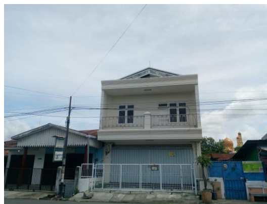
Figure 3. Example of a Detached Building (Two-Storey Residential House)
