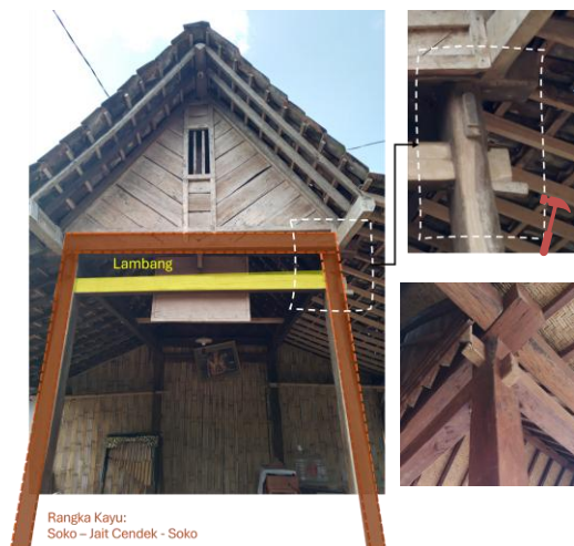
Figure 6. The fastening of Soko - Jait joint (source: author)
