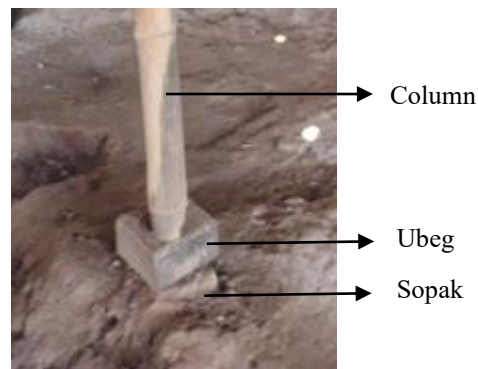
Figure 3. The connection between ubeg and sopak stone (source: author)
