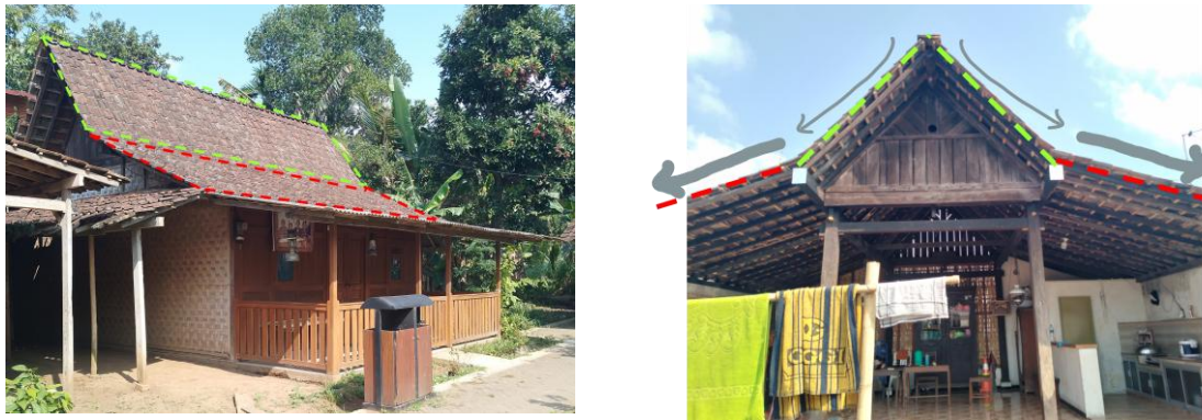
Figure 8. The two segments of the Tikel Balung Roof (source: author)
